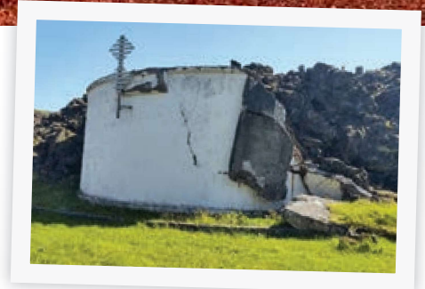
A preserved ruined water tank near the harbour area, half submerged by lavas
