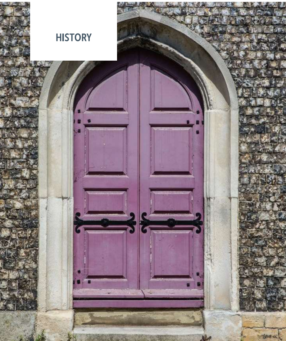
The 1748 exterior wall of St Michael in Lewes Church, Sussex, with finely coursed knapped flint
